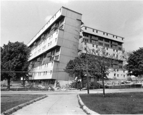
Hartford Park Failed Demolition 1989
